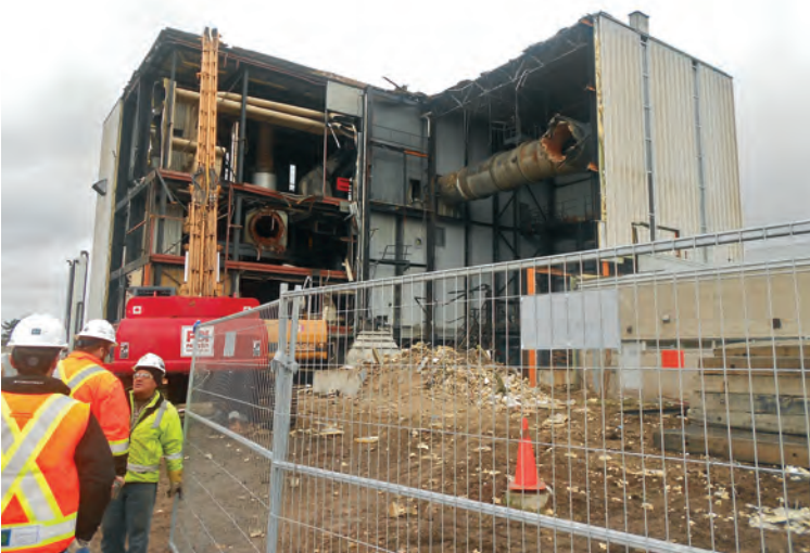
Woodward Avenue Water and Wastewater Treatment plant is getting a makeover.
