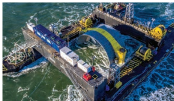
Cape Sharp Tidal lowers its tidal turbine into the water at its Bay of Fundy test site near Parrsboro, NS.
