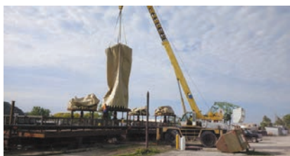
Hydrostor prepares to install one of the air accumulators in Lake Ontario. PHOTO: TORONTO HYDRO
