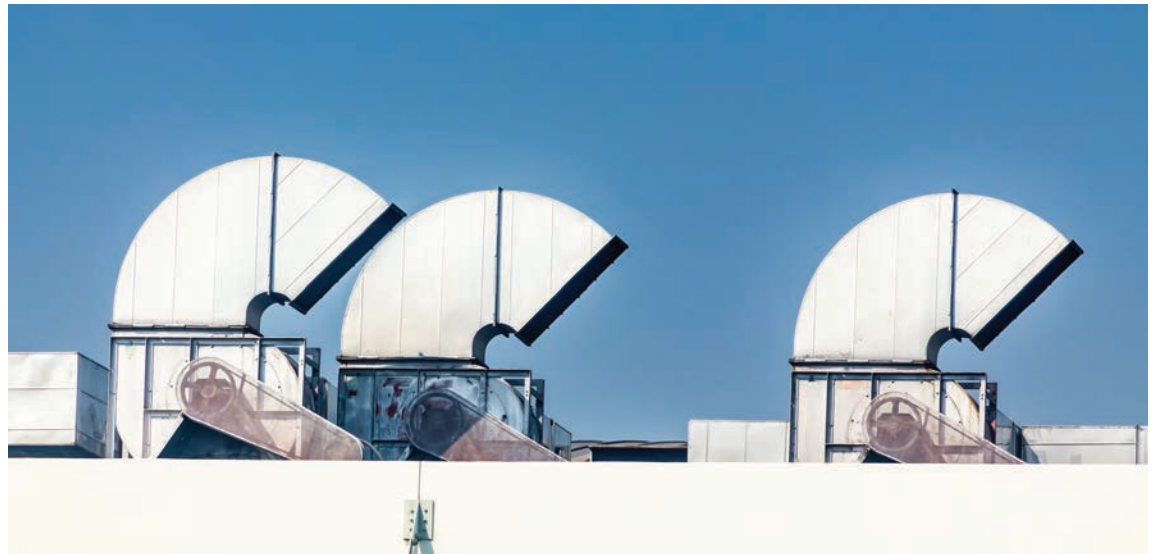
Industrial air conditioning and ventilation.
