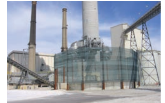
DustTamer wind fencing at a gypsum plant. PHOTO: DUST SOLUTIONS
