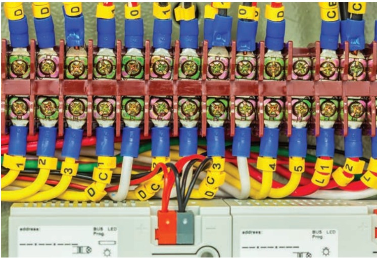
Ensure safety audits and emergency stops are working correctly.
