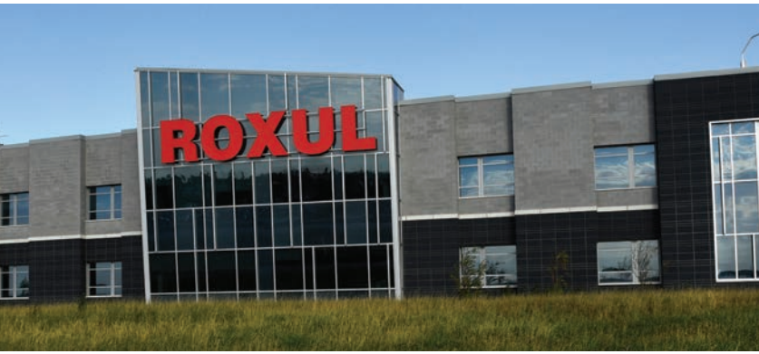
Roxul's Milton, Ont. headquarters.
