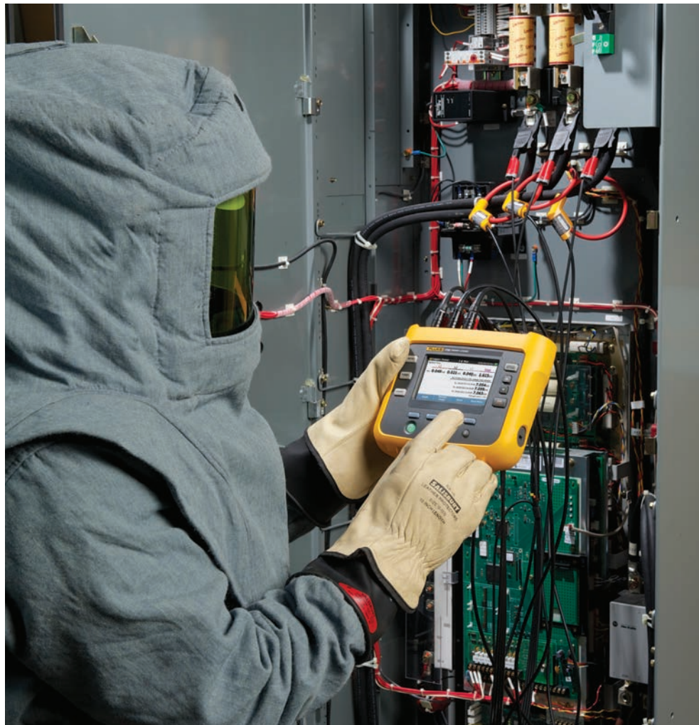
Monitoring power systems to support energy saving initiatives.
