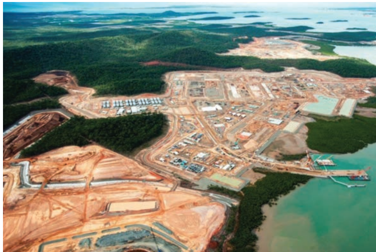
Workforce housing on Curtis Island, Australia.
