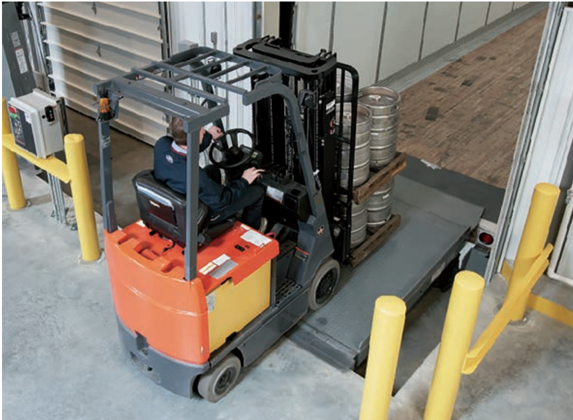
Vertical levellers provide a smooth path between the plant and trailer.
